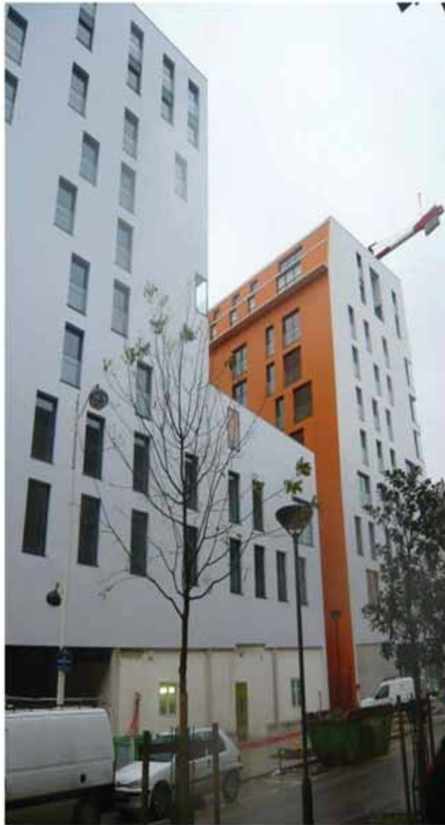
A building cannot exceed 45meters without being interrupted by a void of 8meters minimum
