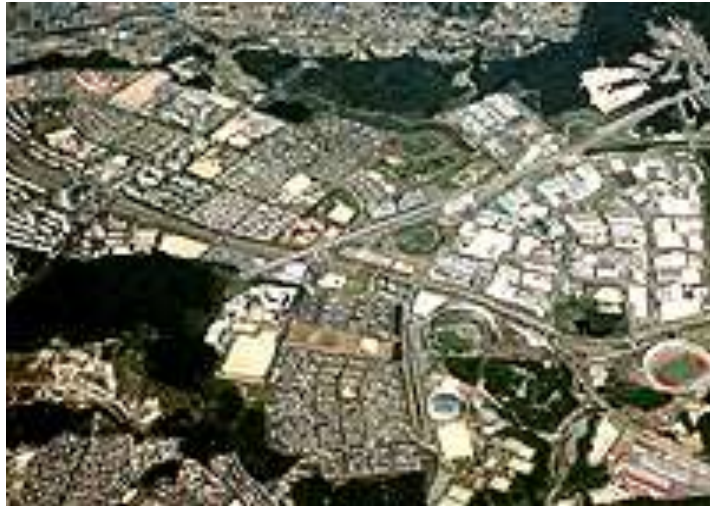
ΚΟΒΕ DISTRIBUTION CENTER
