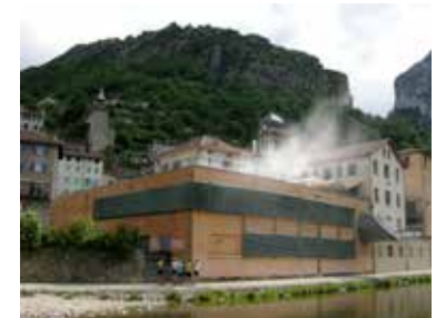
Water Museum (Pont-en-Royans, France)
